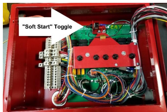
Interior view of engine gauge panel. Figure #3-3
