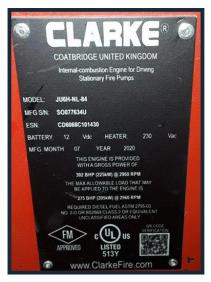
This nameplate shows UL and FM listed certifications on a non-listed engine model.
