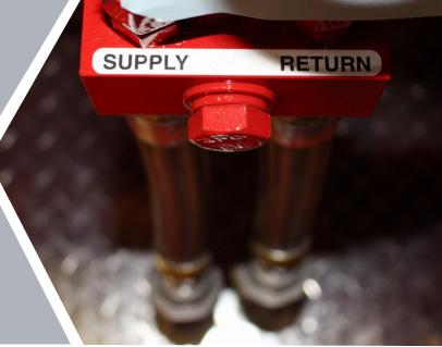
Fuel is one of the 3 key components to make your diesel fire pump driver run. The engine must be equipped with quality fuel hoses used to isolate engine vibration from the fuel lines and fuel tank. These hoses are essential to provide enough fuel to power the engine while having the ability to stand up against wear and tear of regular usage and corrosive environments.
